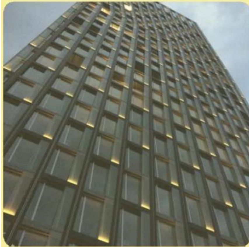
Preferred Exterior lighting
